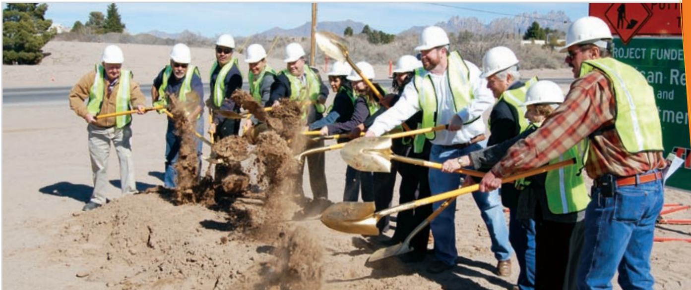
Groundbreaking for Del Rey Boulevard improvement project
